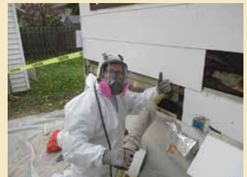
Weatherization Specialist installing exterior wall insulation
