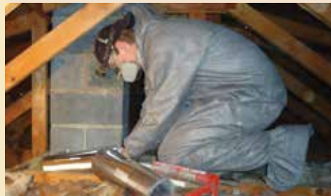
Making improvements to client's attic
