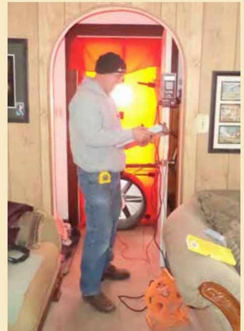
Blower door testing being performed by an ADVOCAP Field Technician.
